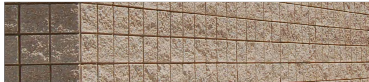
Existing: Tile Building Entry & Wainscott
